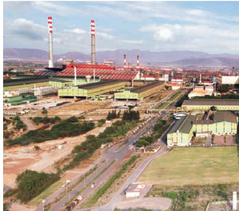
Panoramic view of Vijayanagar Works
